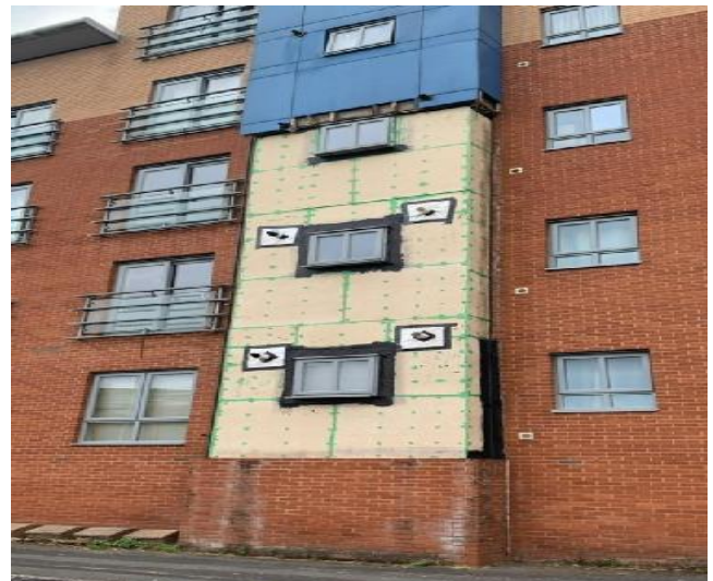
Progression on Elevation B4
