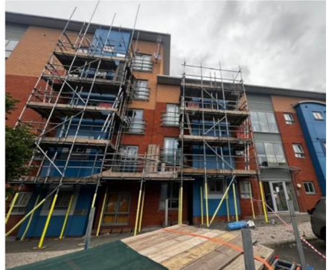
Progression on Elevation B
