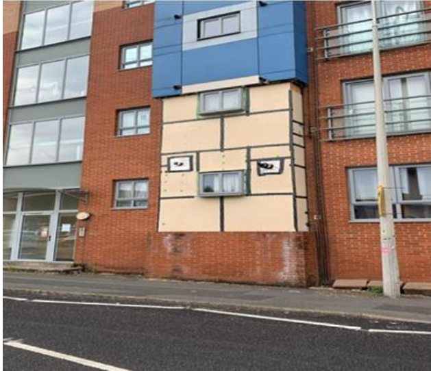
Progression on Elevation B2
